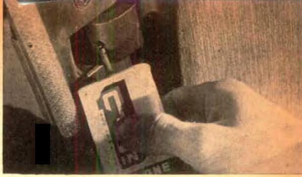
**Concealed hinges** are oiled from the inside of the open door. Close examination will usually disclose an oil hole in the hinge.
