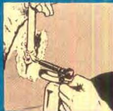
Good tinning is essential. A thin tinning coat is first flowed on and then scoured with steel wool to provide an anchor for the solder.
