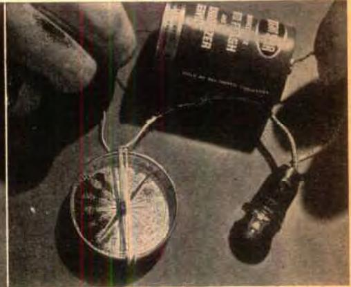
bulb, needle will swing to one side, repelled by magnetic field set up in coil. Now switch connections to battery, reversing direction of current flow, and needle will swing other way. This is what happens in car's ammeter. When battery is charging, current flows one way; when discharging, current reverses.
