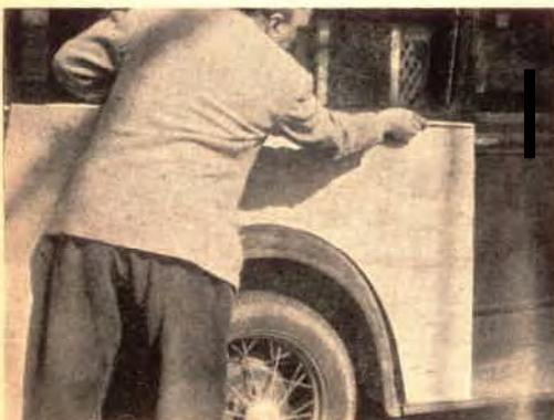
**5** Cap top edges of panels with wood sills, covering space between metal and panels. Mastic in the joints will lessen squeaks. Attach panels with  $\frac{1}{4}$ " rustproof bolts.
