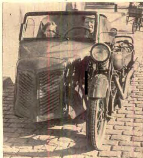
WHEN August Paul travels with his motorcycle, he rides comfortably in the sidecar instead of straddling the bike in conventional fashion. A mechanic in Munich, Germany, Paul rigged up the vehicle himself, installing a steering wheel, gear shift, and other controls in the sidecar.
