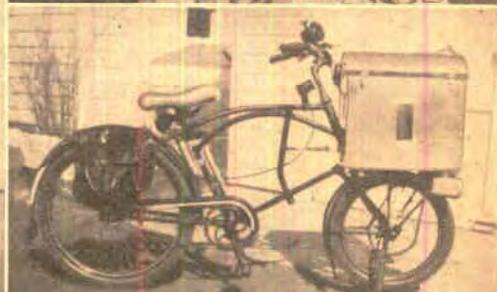
**Front Wheel Is Motorized.** Using a standard bicycle as a base, Dr. William S. Voorhees constructed this unique front-wheel driven motorbike. In addition to the 2-hp. engine, the front housing holds a 1-gal. gasoline tank—enough for 120 miles. The motor is connected through a belt and a ball-bearing idler pulley to a countershaft
