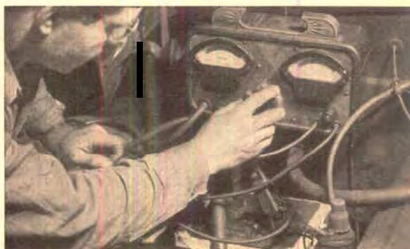
**2. Good ignition** depends on a battery in good shape. Here each cell is being checked under load. Corrosion is removed from terminals and cables examined.
