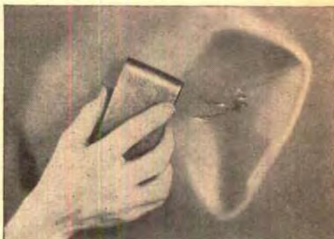
**Short, tight jams** take hammer work from inside and a bumping dolly against the outside. Again confine the blows to the edges.
