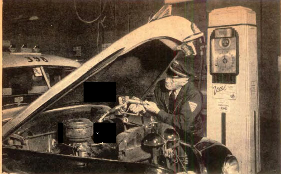
**Water injection** is another way of conserving gasoline quality. In Cleveland, Yellow Cabs are now making a wholesale test of the Vitameter  $\text{\textcircled{T}}$ , an injector developed by the Thompson Prod-
