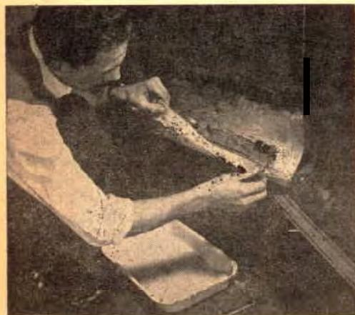
**5. Successive layers of Celastic <sup>®</sup> may be used to build up spots where the original metal is completely gone.** Allow each layer to set 15 to 30 minutes before applying the next one.
