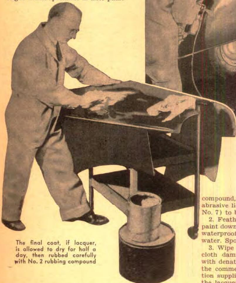
The final coat, if lacquer, is allowed to dry for half a day, then rubbed carefully with No. 2 rubbing compound
