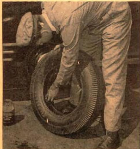
Mount the tire on the rim, inflate to recommended pressure to seat the beads, deflate, and reinflate.
