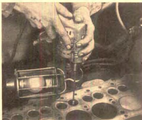
**10. All valve guides** are cleaned with a reamer chucked in the ever-handly drill. Sometimes, a guide is worn so much that it must be replaced. Note the clean block after the carbon removal.
