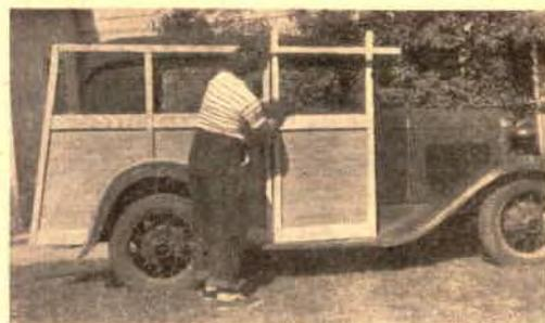
**8** Leave top longitudinal of rear panel over-length to serve as guide in fitting the door panel. Clamp the latter in place to try it. Allow at least  $\frac{1}{2}$ " clearance over the running boards so snow or ice won't jam the doors.
