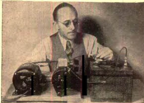
**1** The complete unit, consisting of a shop motor, an old generator, a cutout, and an ammeter, is pictured here in finished form, charging an automobile storage battery
