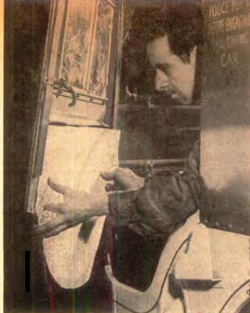
As a stiffener, the fabric may be used in many ways. At the Crystal Collision Co., Brooklyn, it's applied inside aluminum cabs on Jeeps  $\text{\textcircled{T}}$ .
