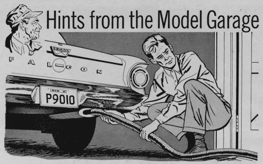
Make your garage a safe place to work in when you tune up your car's engine by venting deadly carbon monoxide exhaust gases outside with a snaking tailpipe extension. A length of flexible steel tubing or an old vacuum-cleaner hose will do the job. Be sure the diameter of the extension is such that it makes a leak-free fit around the tailpipe. Run the free hose end outdoors—and away from windows and siding: Exhaust fumes can discolor painted woodwork and corrode exposed metal surfaces.
