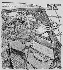
Weatherstrip that freezes to the door jamb after snow or sleet is often torn loose when you pull open the door. This won't happen if you clean the rubber when it is dry and coat it with brake fluid or rubber lubricant.
