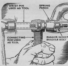
Wrist Pin Drives Shackle. When installing rubber-insert shackle bolts, George Pedley, of N. Grosvenordale, Conn., uses two other parts as tools. A wrist pin, annealed by heating, is employed for driving the bolt, and a connecting rod is used as a guide to keep the rubber from expanding.
