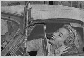
A SPEED-LIMITATION HORN for gas-and-rubber-saving drivers, toots its warning when the speedometer needle makes contact with a button set at the 35-mile mark on the dial. Contact opens a valve in the exhaust, which in turn blows the horn.
