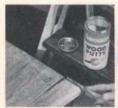
Step 2. Rebuild broken corners, fill micks and holes. A powder-form plastic putty, Savogran Wood Putty, is ideal for this. You can form it, tool it . . . and it doesn't shriak. For cracks in plaster, use Savogran Crack Filler. It's the original patented quick-hardening water putty.
