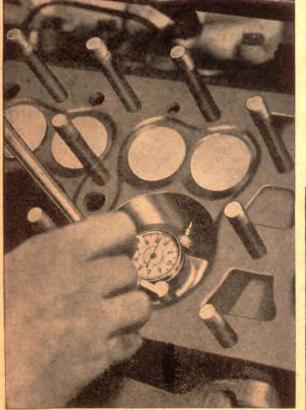
CHECKING THE CYLINDER BORE will show whether honing is advisable. Here a dial gauge is used. Right, a typical piston with its parts named
