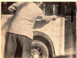
5 Cap top edges of panels with wood sills, covering space between metal and panels. Mastic in the joints will lessen squeaks. Attach panels with K" rustproof bolts.
