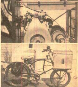
which is geared to a sprocket on the front wheel. A brake on the countershaft is actuated by a handlebar lever; with this and the coaster brake, both wheels have braking action. Speeds from 6 to 42 m.p.h. may be obtained, and the bike is said to be quite stable on turns as well as straight runs. The speedometer works off the rear wheel.
