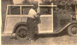
8 Leave top longitudinal of rear panel overlength to serve as guide in fitting the door panel. Clamp the latter in place to try it. Allow at least £" clearance over the running boards so snow or ice won't jam the doors.
