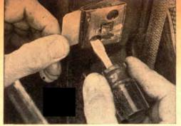
Worn-down latches are adjusted quickly with a metal shim set in behind the strike. Loosening the screws will permit inserting the shim.
