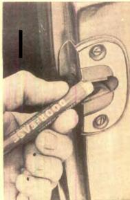
Jamb strikes require lubrication with stainless graphite, which may be had in the convenient pencil shape. The strike shown has rubber insets that can be replaced by removing the two screws.
