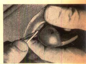
Take off door handle and window crank. Press inward on base plate to expose lock pin. Use small nail to push pin out of collar and shaft.
