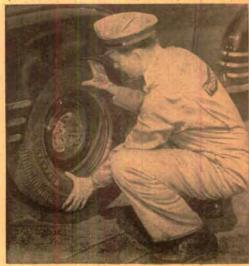
Make sure there is no grit on the tube or inside the casing. Insert the tube, inflate until it is nearly rounded out, and replace the valve cap. Photos by Firestone
