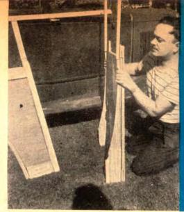
7 Cut the inside panel frames to follow the contours of original body. Remove handle from door for greater ease in fitting door panel. In stage shown above, rear panel is assembled but has not yet been attached permanently. Be-
