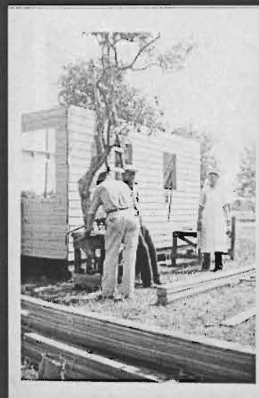
Turner, Dick & Ches Cutting roof boards (Note meat saw)
