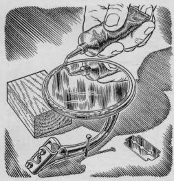
If a mirror rattles in its frame, transparent windshield-glass sealer or a clear cement applied between the glass and rolled edge will keep it quiet. Remove mirror and place it flat to do the job. Scrape off excess cement with a razor blade.
